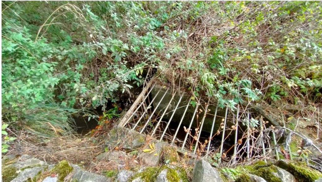
Figure 2: Grill on upstream end of Culvert, Dirty Lane.
